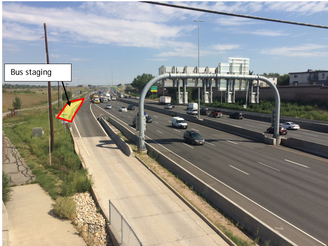
Figure 29 - On 88th Ave looking north on 8/23/17 around 10:30am
