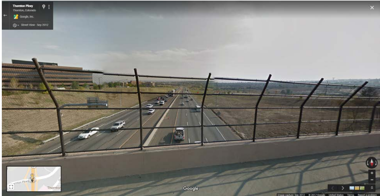
Figure 9 - On Thornton Pkwy overpass looking south (2012 Street View)
